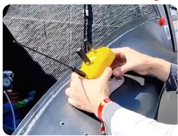
Allow for 10cm of cable lift available (A "Fist" underneath)
